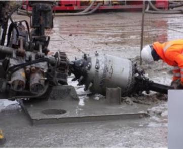
End of directional drill reaming bit appearing from the bore
